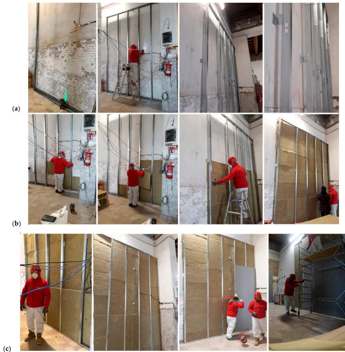
Figure 4. Installation of the selected insulation system.
