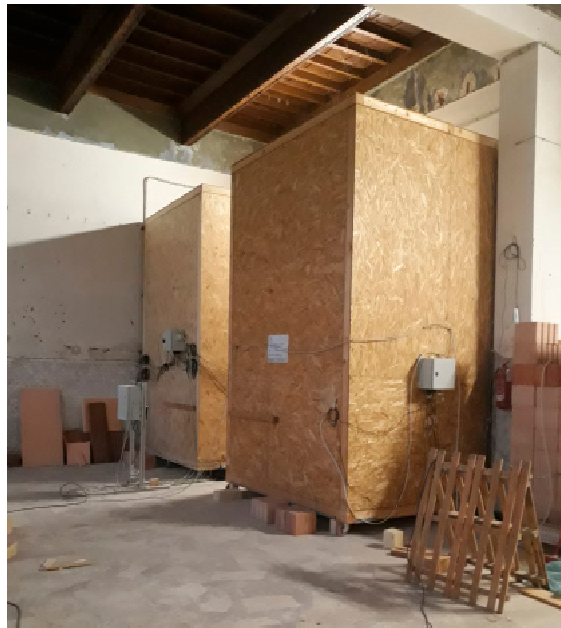
Figure 5. Internal view of the room, with the two boxes tied up to the studied wall.
